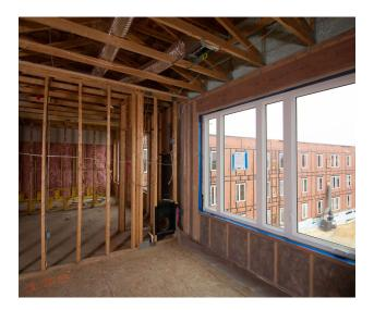
With excellent thermal and acoustic performance, Owens Corning® PINK Next Gen™ Fiberglas™ insulation was an ideal choice for a family-friendly development. The product is fire- and mold-resistant and is offered in numerous R-values to adhere to Wisconsin's specific codes that specify unique insulation requirements based on where it is installed on the structure.
